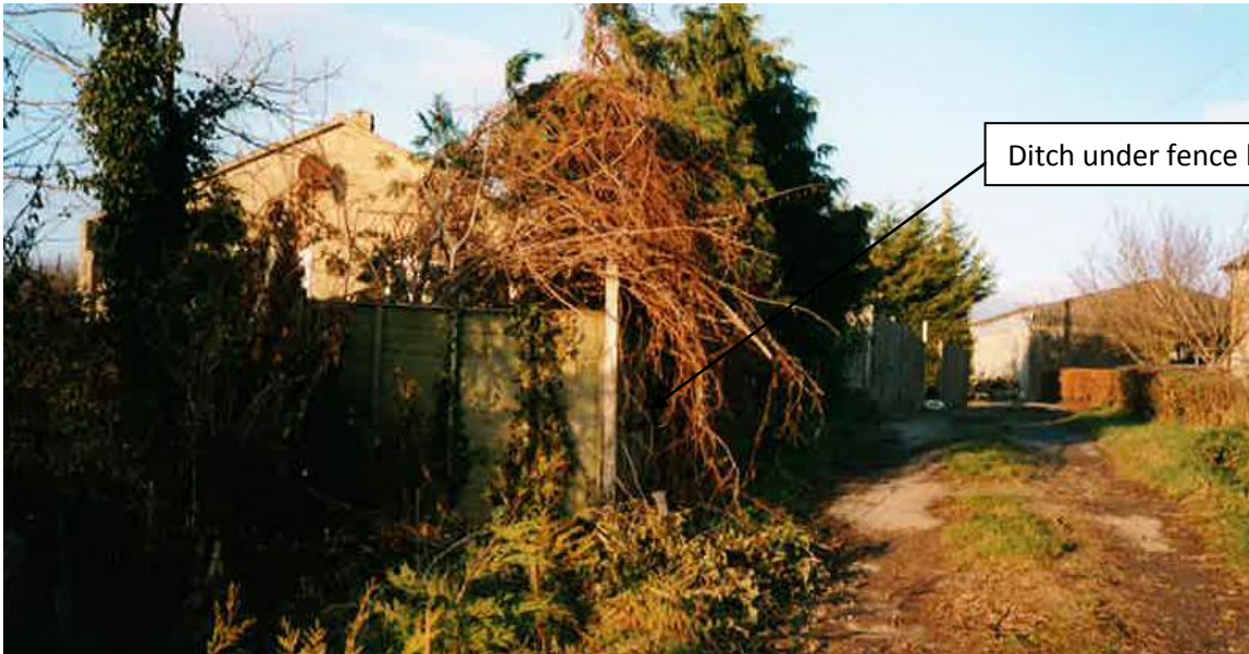
Close up of fencing and piped ditch
